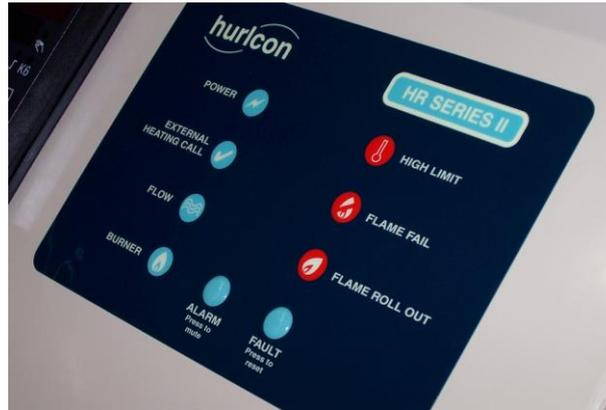
Alarm mute and fault reset buttons are located below the led indicators. A high limit fault will also require the high limit safety thermostat to be reset located on the front of the main electrical panel.
