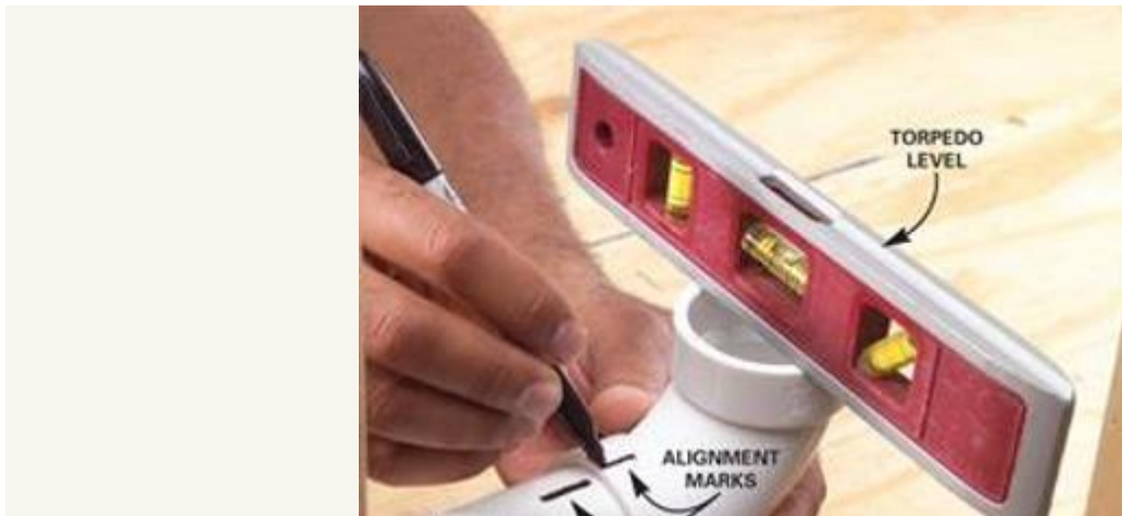
Photo 1: Mark the pipe and fitting
